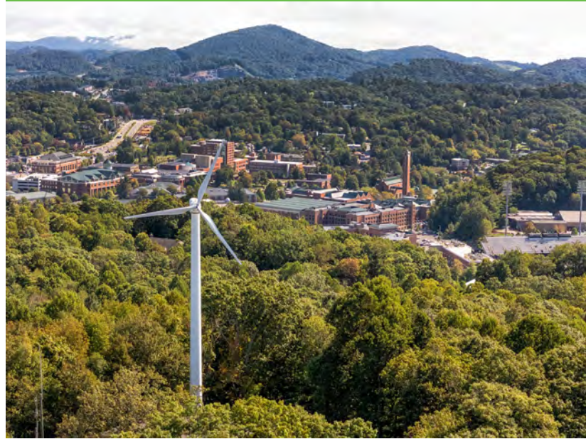
Wind turbine at Appalachian State University.
