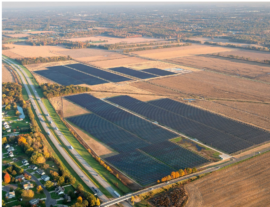
Aerial view of the Notre Dame St. Joseph Solar Farm. Photo credit: Barbara Johnston, University Photographer
