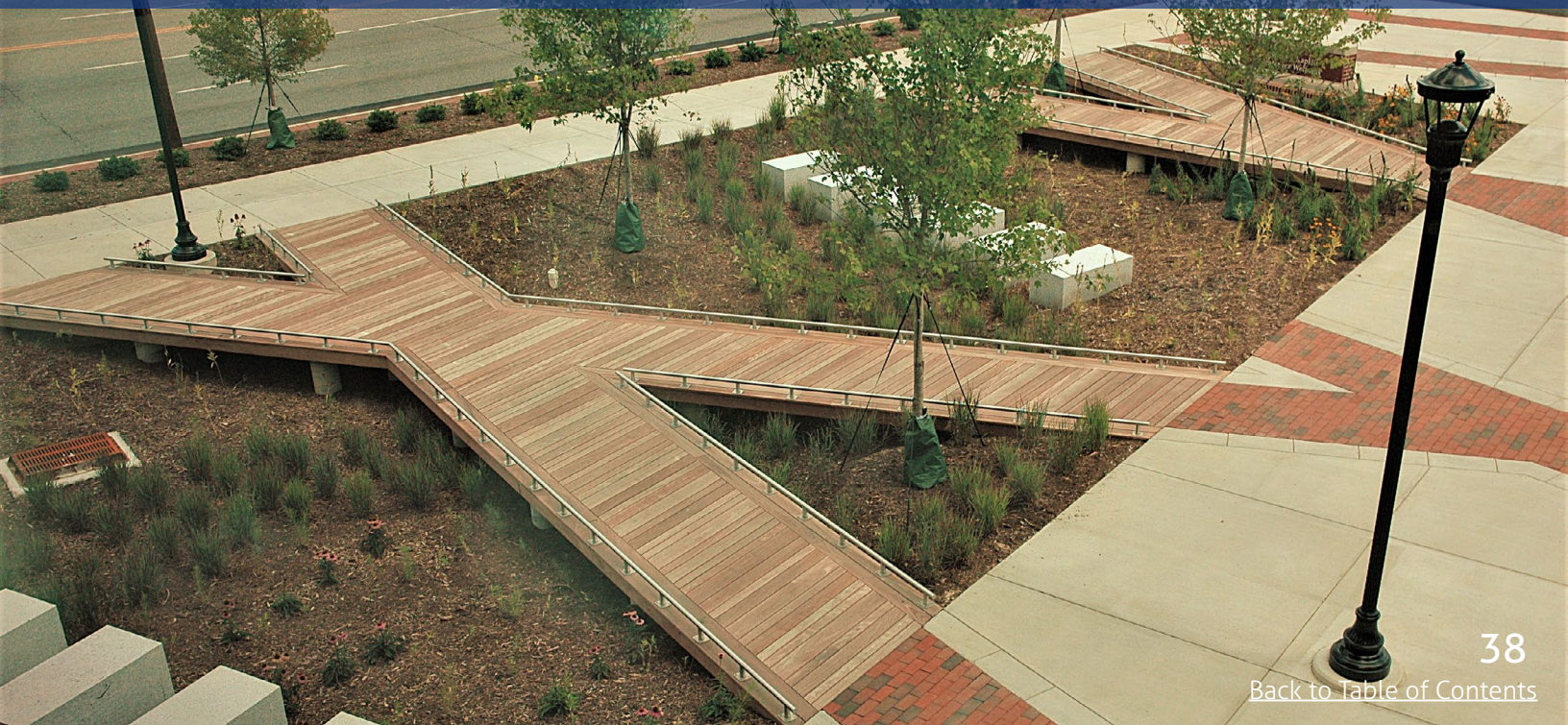
Bioswale stormwater biofiltration system at UNC Greensboro. Courtesy of University of North Carolina, Greensboro.
